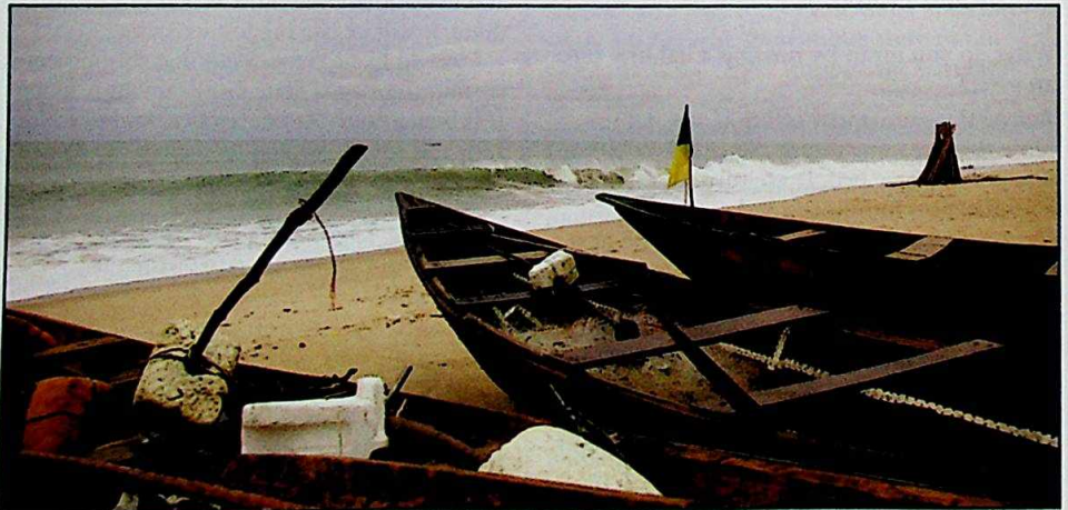
Sea defence walls and other measures have been put in place to protect the beaches and ports of Lagos from the surges of the Atlantic Ocean.
