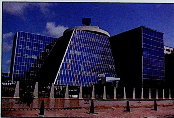
Lagos is home to the Nigeria Stock Exchange and is the base for 200 listed firms. The headquarters of First Inland Bank reflect a positive vision for the future.
