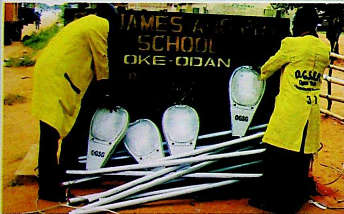
Workers moving equipment to site for Oke-Odan streetlight project.
