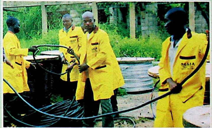
OGSEP workers laying cables for streetlight project.
