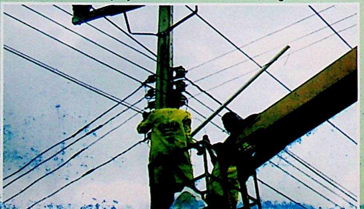
OGSEP workers working on Rural Electrification project at Oke-Ore, Yewa South.
