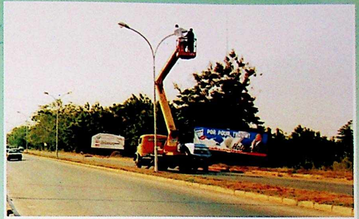
One of the typical sites during streetlighting installations
