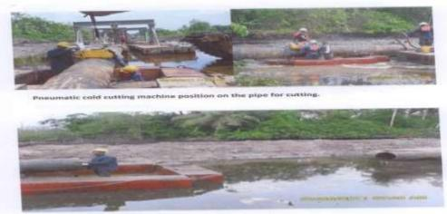
Cut anotion of pipe with work basin (leak point one).
