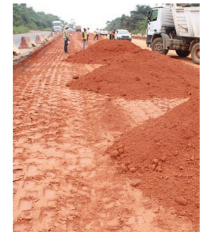
Ongoing Rehabilitation of Lagos - Ibadan Express.
