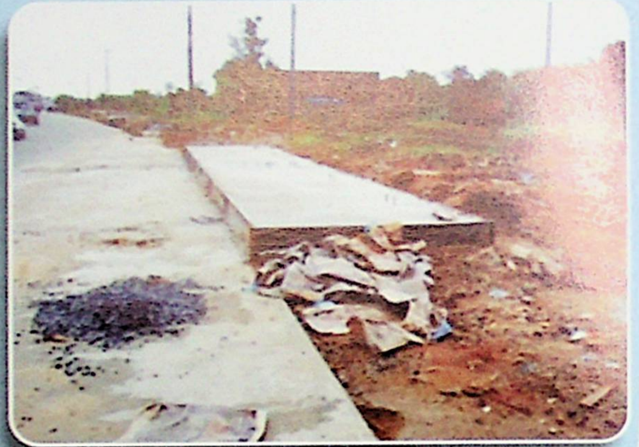
The Platform of the Bus Shelter
