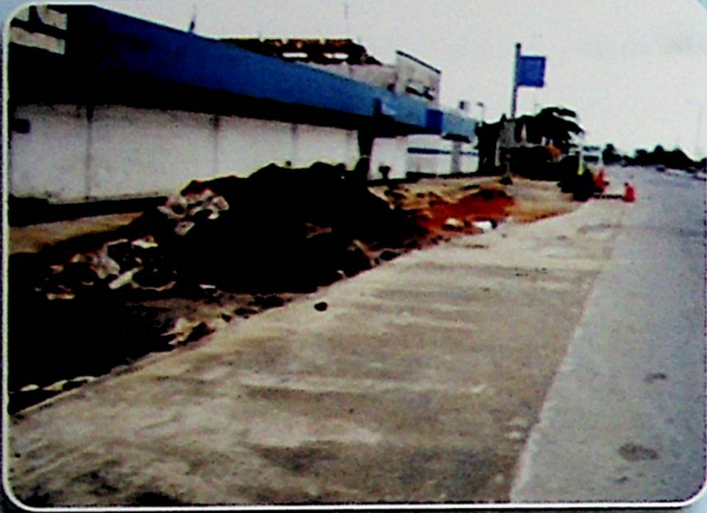
Site Clearing at UTC Bus Stop
