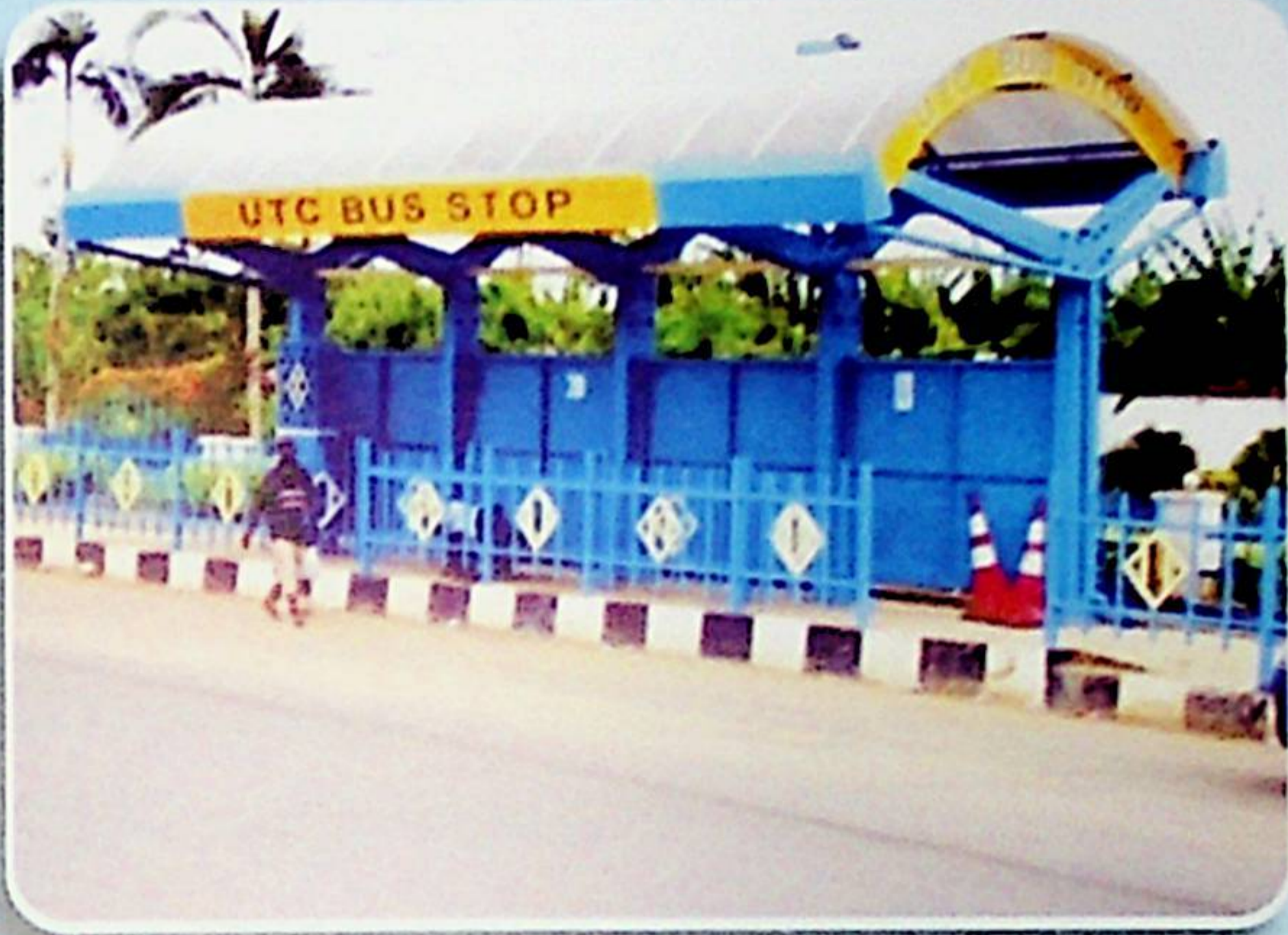
Completed Bus Shelter/Lat-bye at UTC
