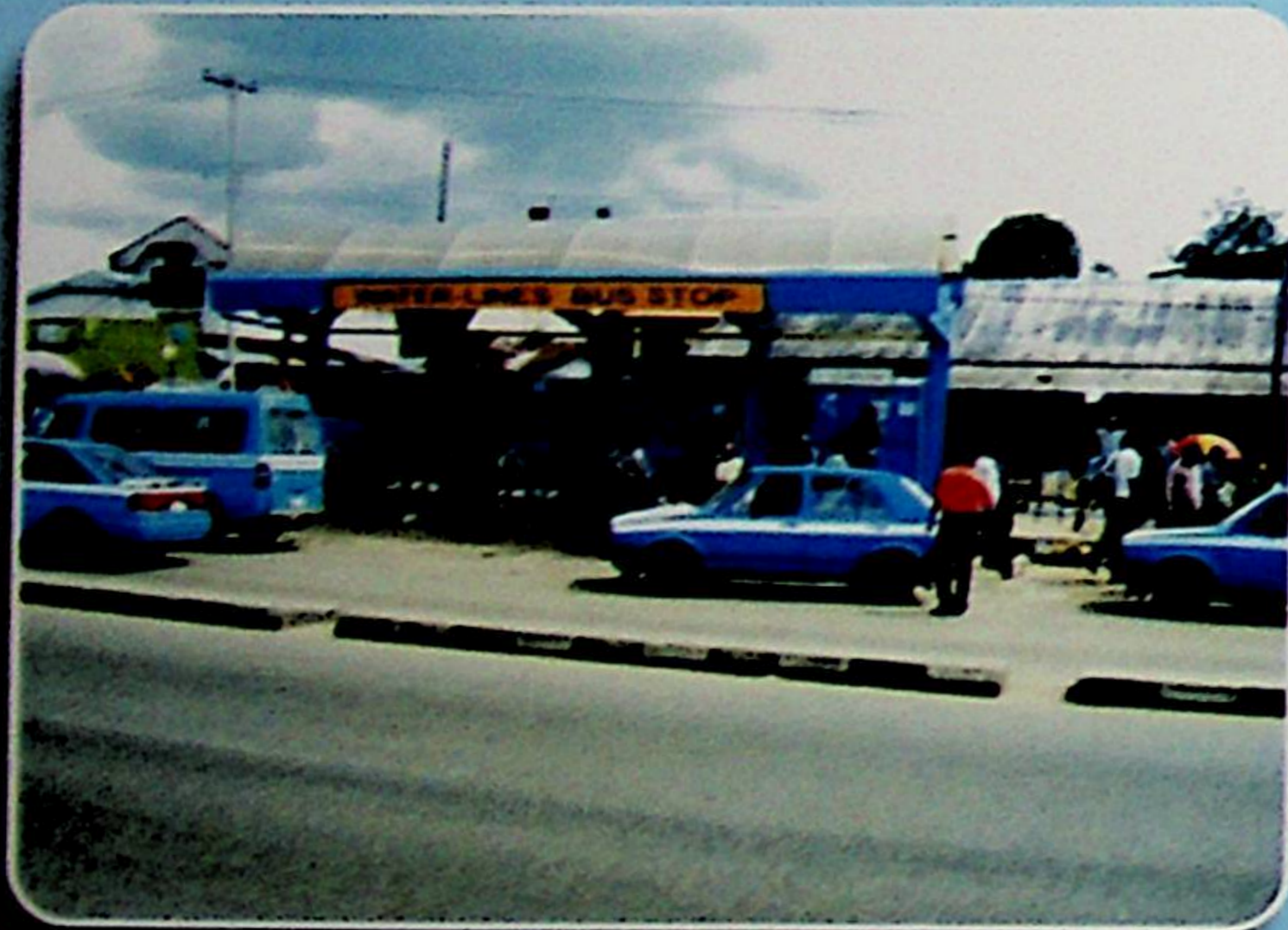
Bus Shelter at Water-lines
