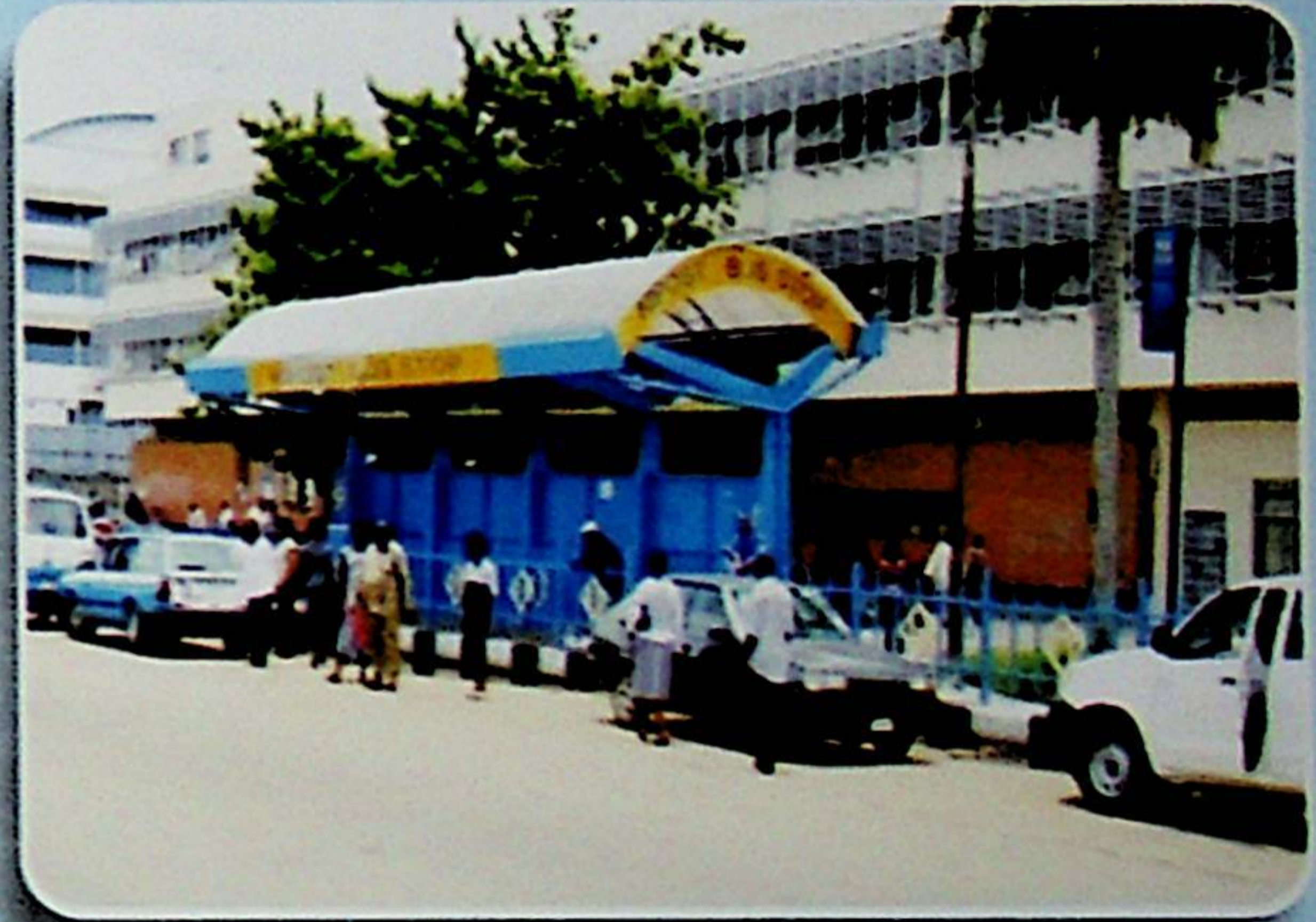
Bus-Shelter/Lay-bye in use at UTC
