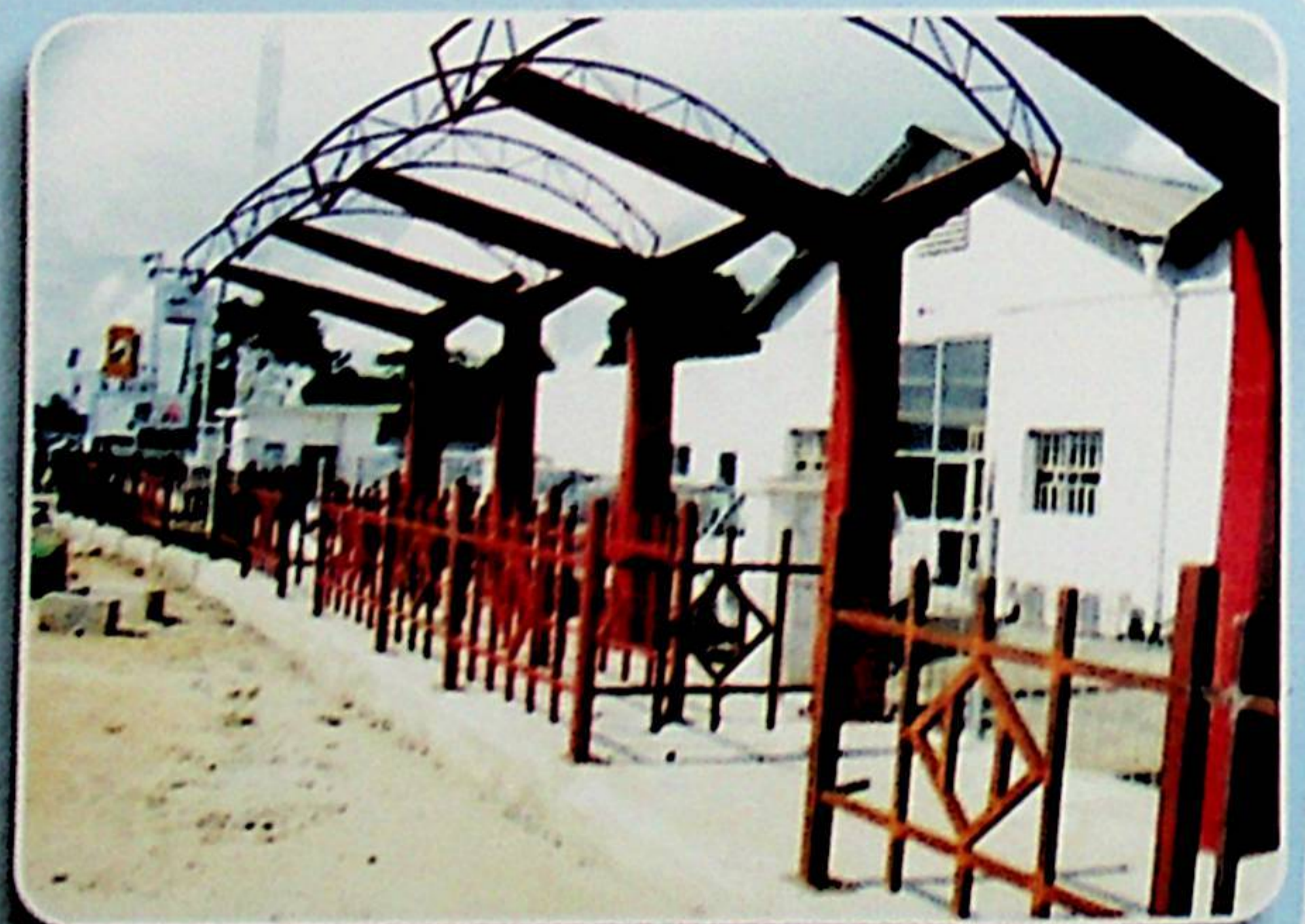
Bus Shelter Steelwork at UTC
