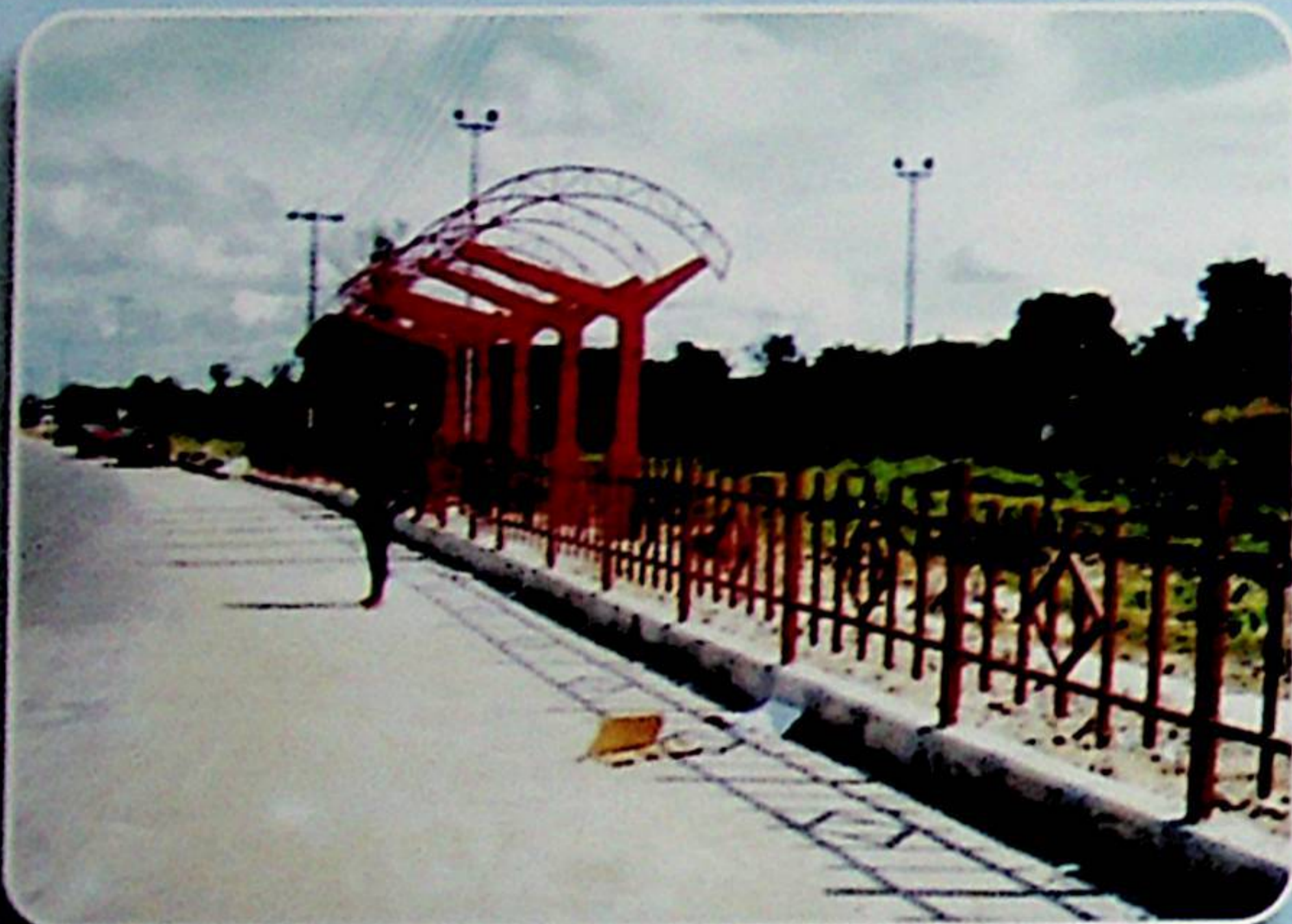
The steelworks for the shelter at NIPOST
