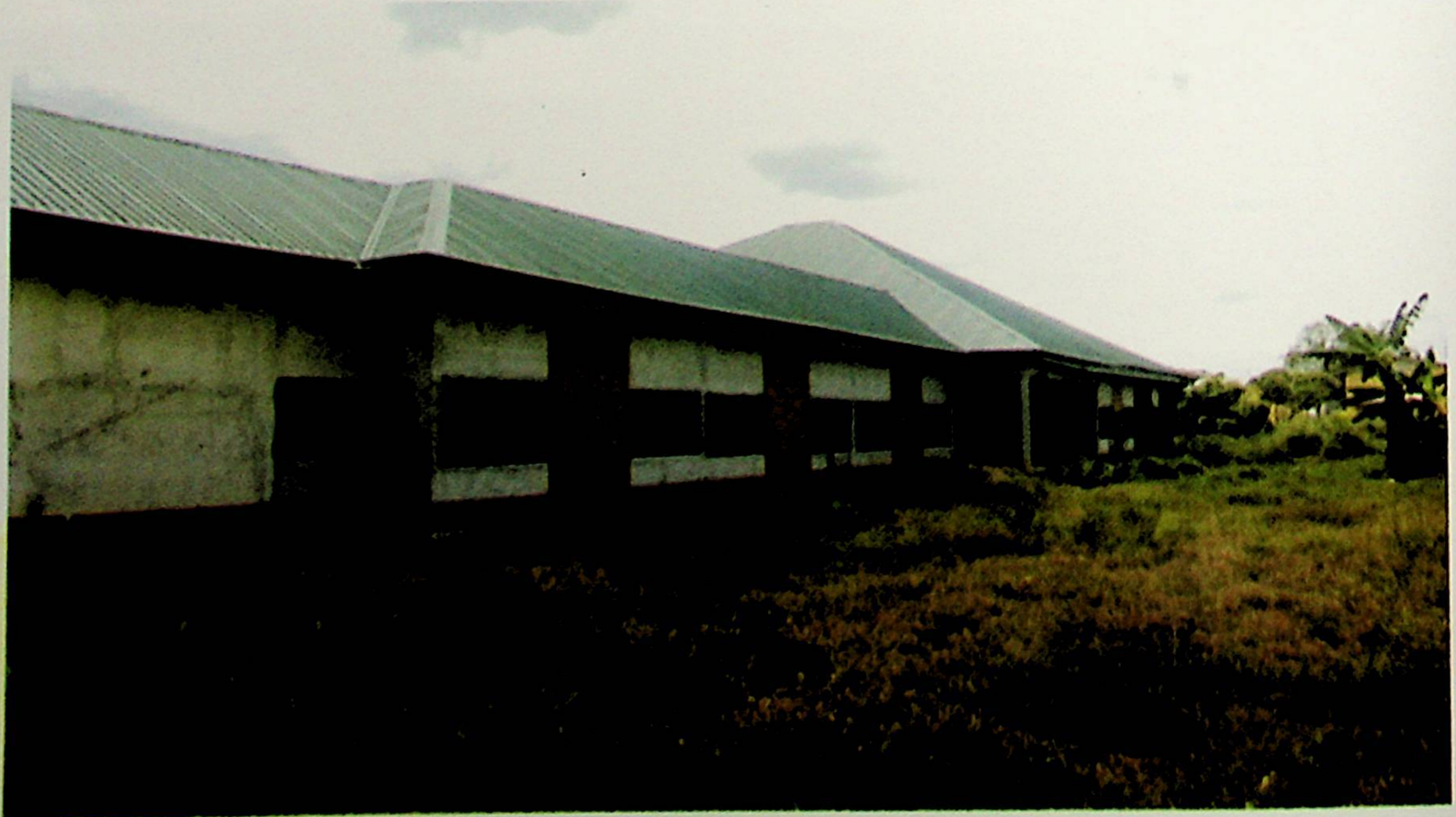
Government Primary School In Ahoada East L.G.A. under construction
