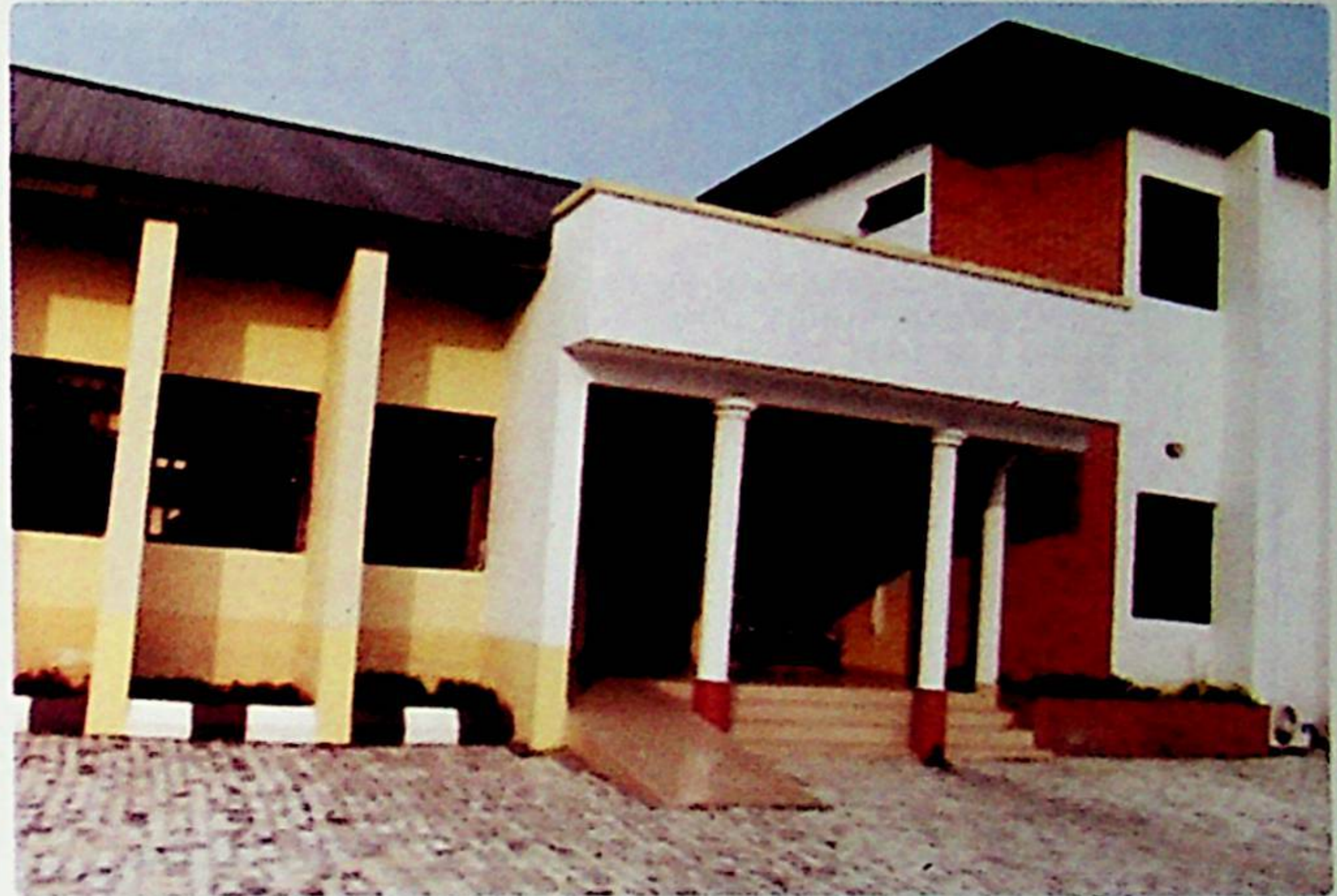
Primary Health Centre, Wiiyaakara
