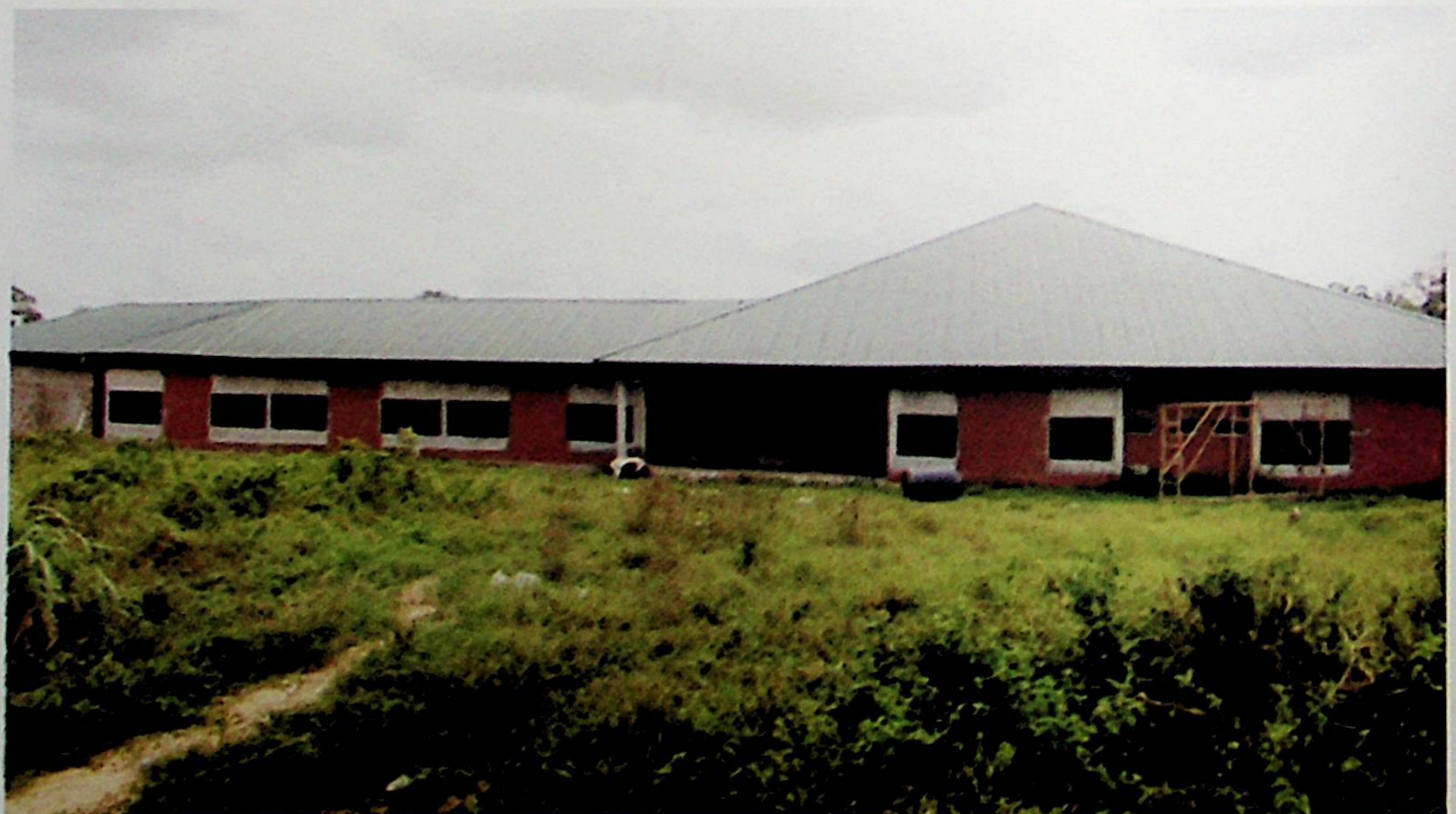
Akinima Primary School under construction
