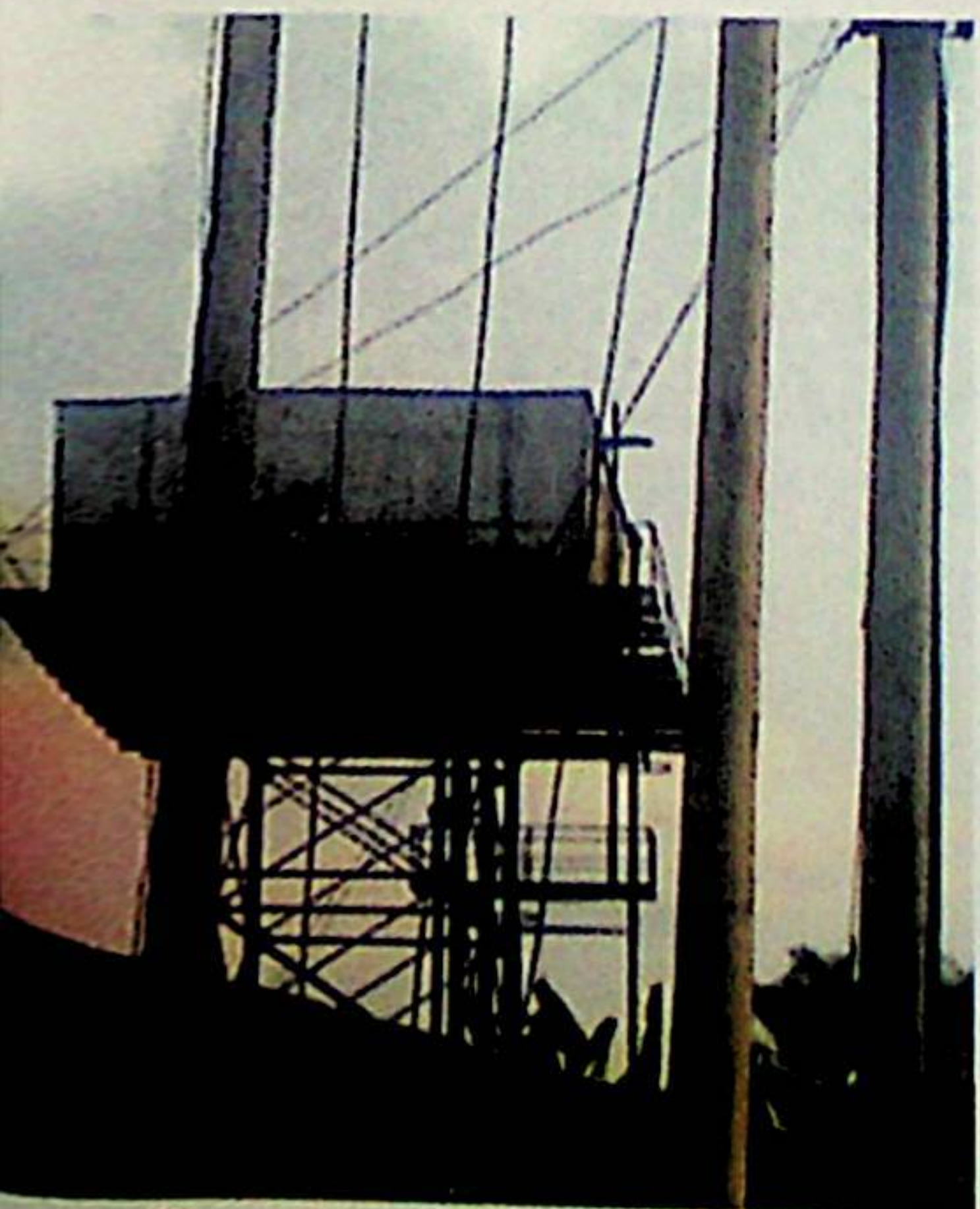
The utility pipe borne water project
