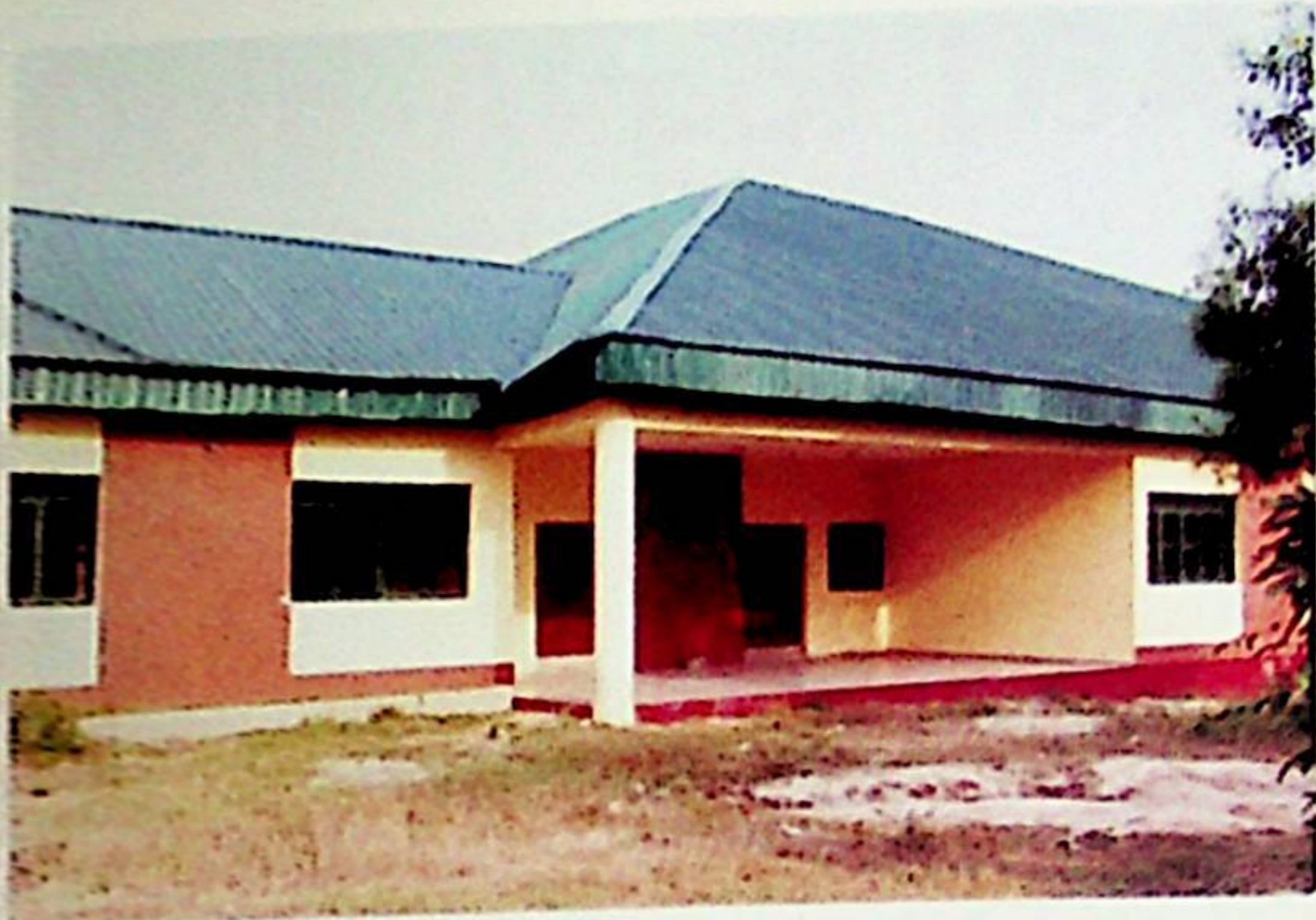
Model Primary School Zaakpon under construction
