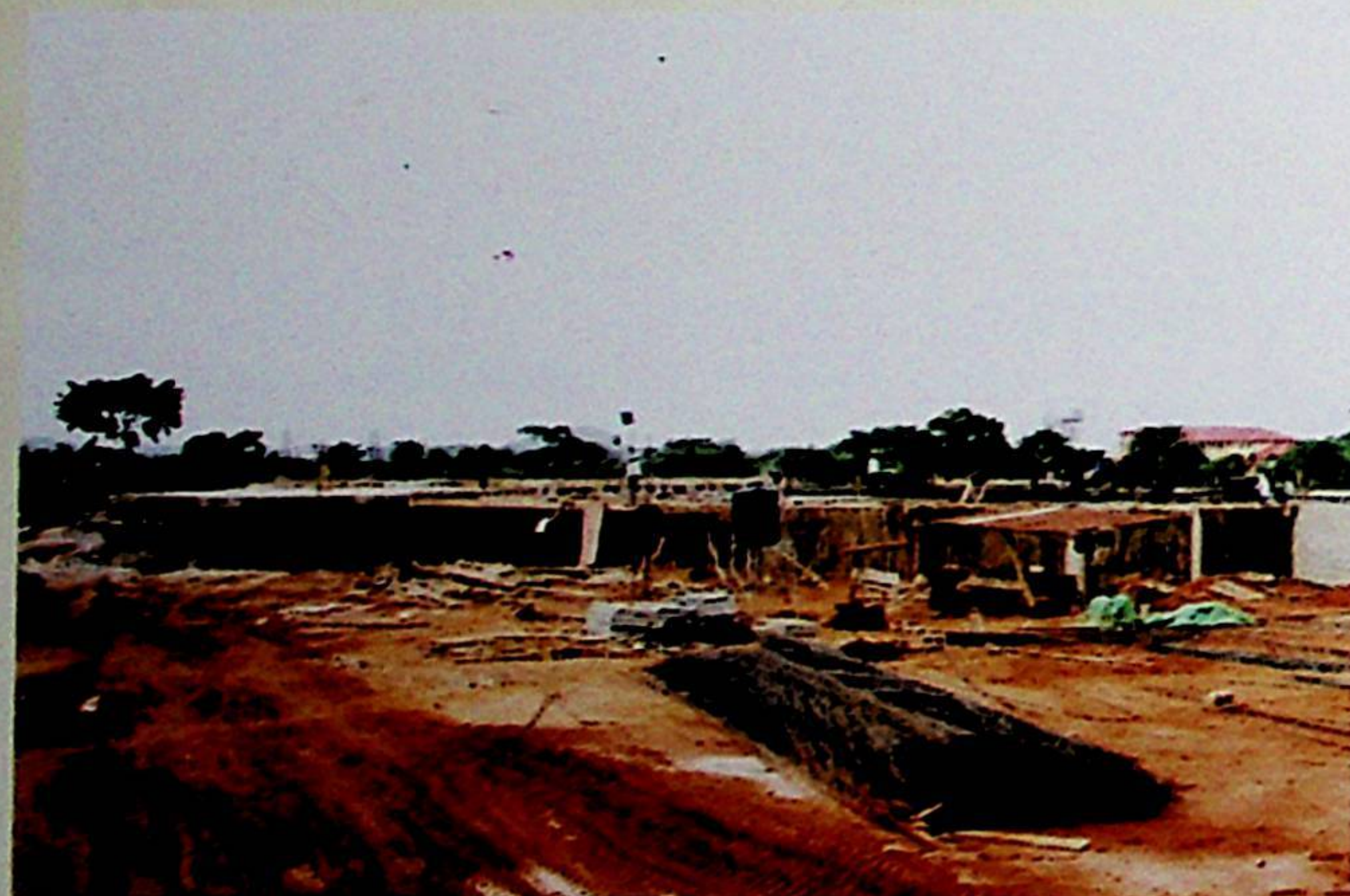
Construction In progress
