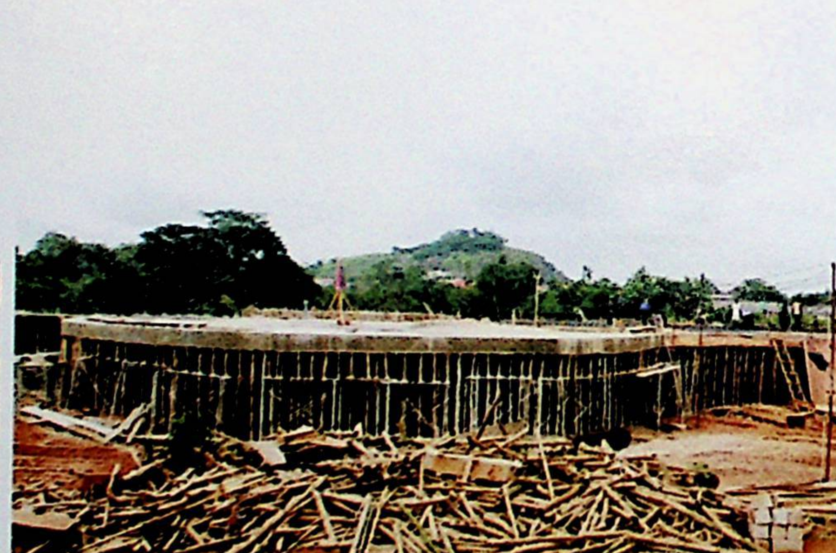
Structure to carry the Dome
