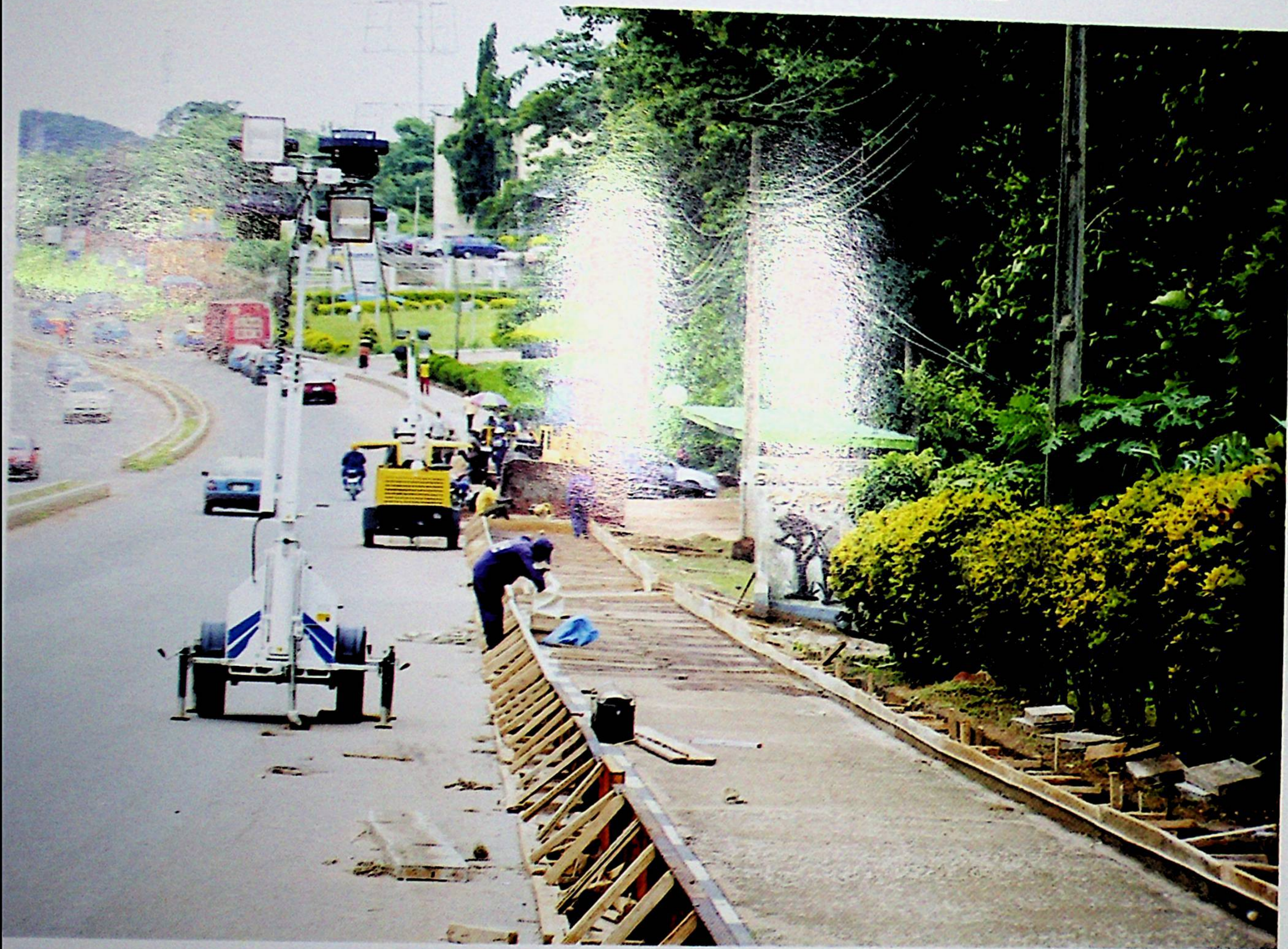
A section of the Oba Adesida road being rehabilitated
