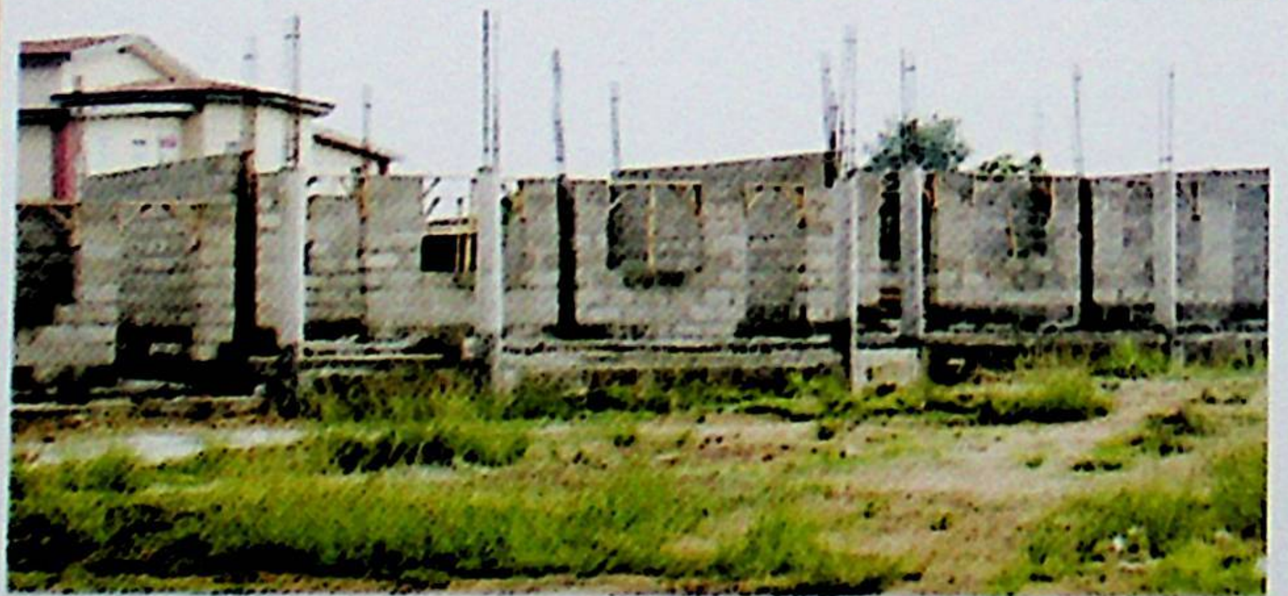
A section of the Caring Heart Mega Primary School under construction
