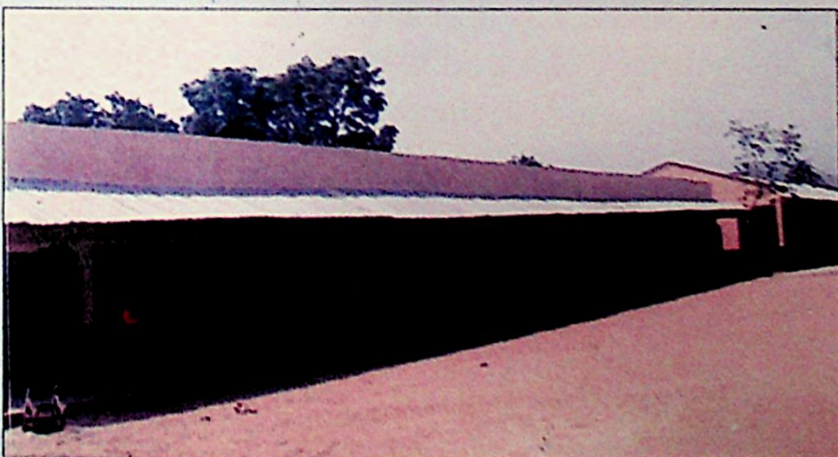
Ofudu School Project (Igalace LA/Odoju LGA)
