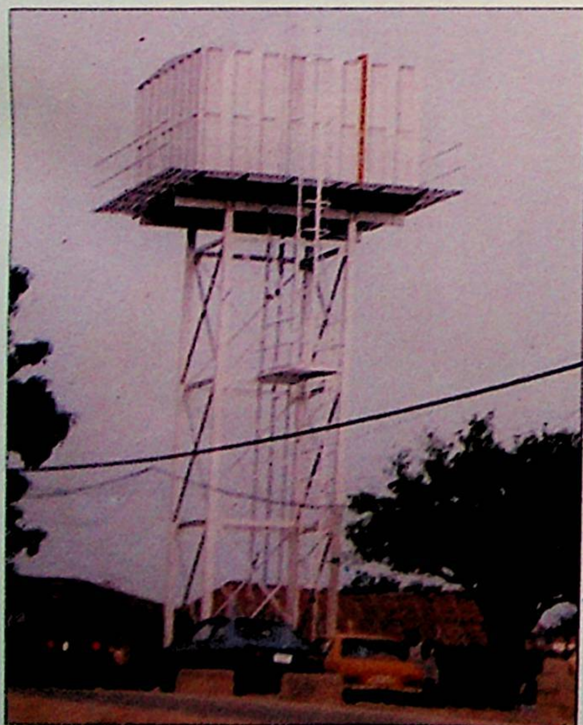
Prototype Motorized boreholes with Overhead Tank
