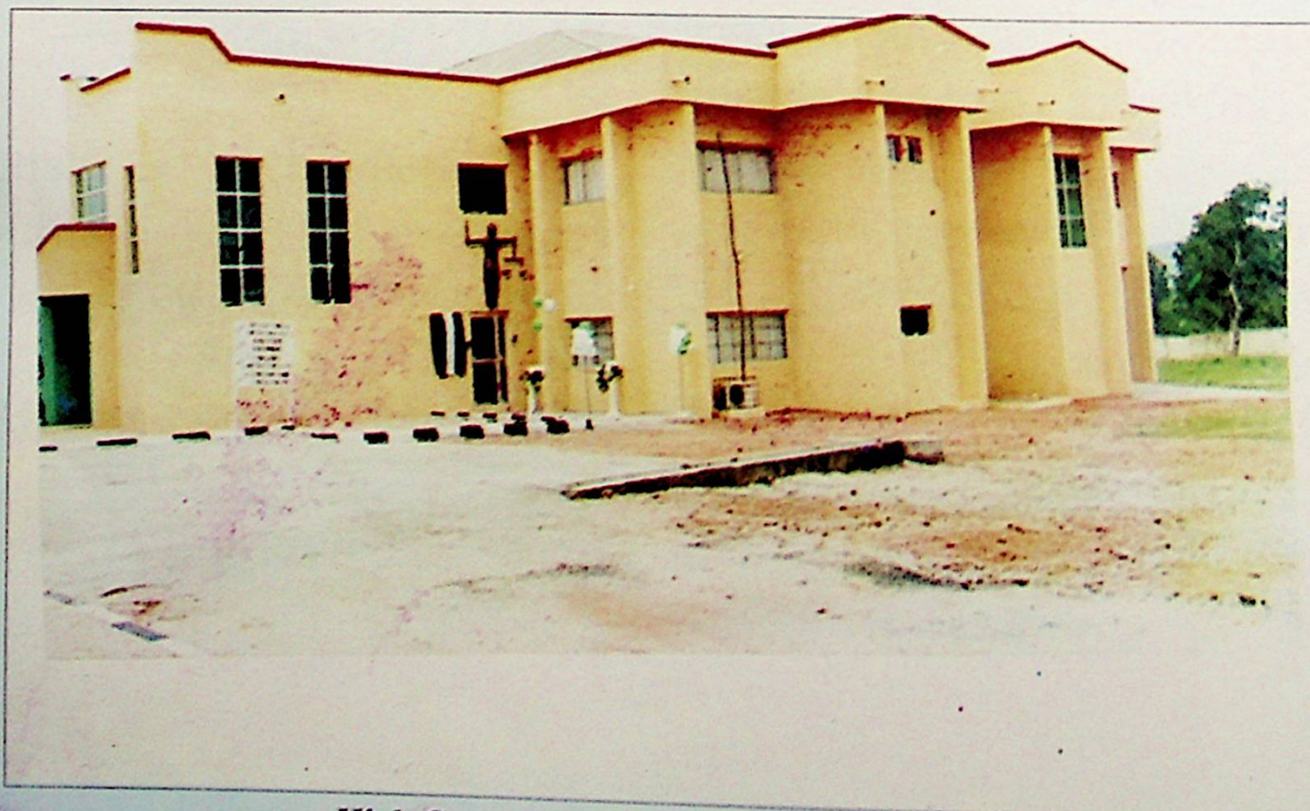
High Court of Justice Extension Project
