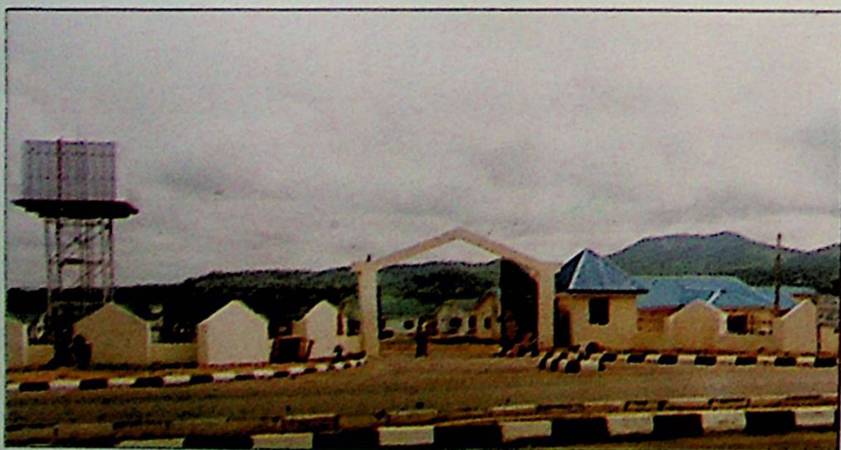
250 Units of 3,2 and 1 bedroom bungalows, Ganaja Road
