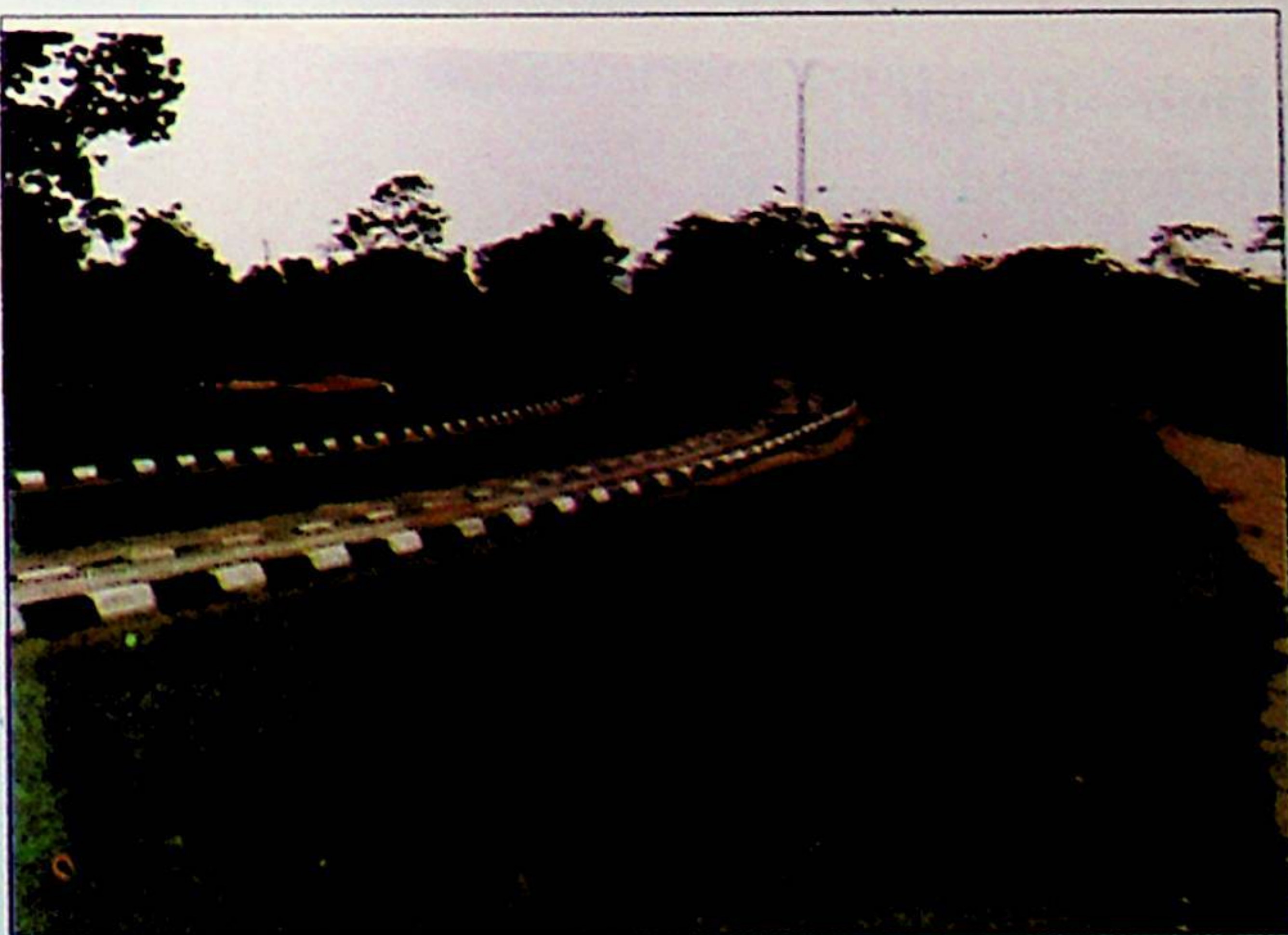
Meme Bridge and Access Road.
