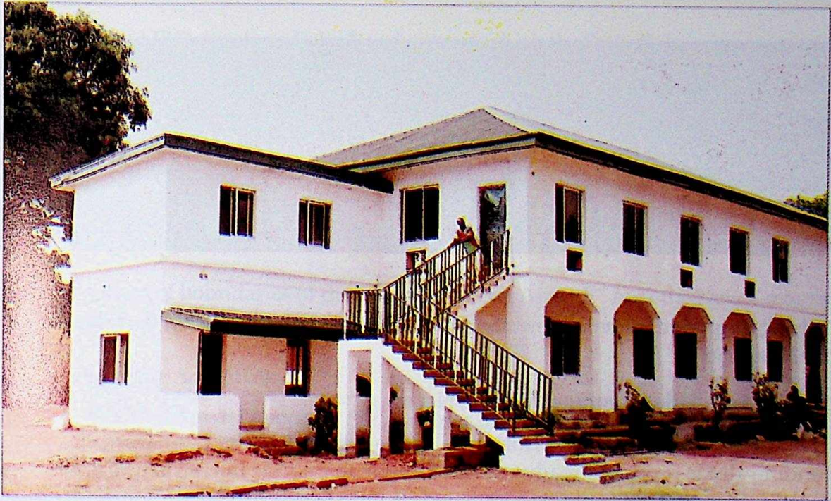
Federal Court of Appeal building at Okigwe Road, Owerri
