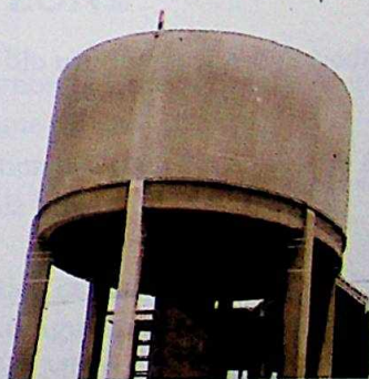
Overhead Concrete Tank at Nnempi Water Scheme
