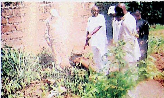
Bore hole at Mgbidi water scheme
