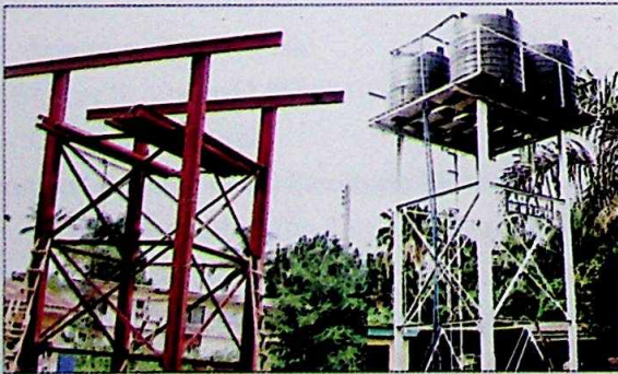
Water Bore Hole Project Okohia, Isiala Mbano
