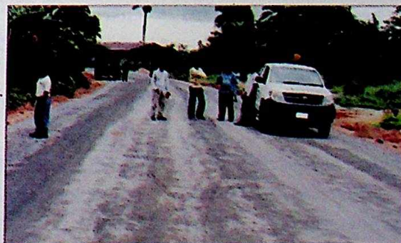
ISOPADEC on-going Road Project at Ogbujiagu Abacheke in Ohaji/Egbema LGA
