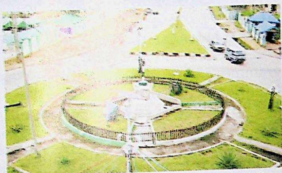
Beautification of Okigwe, Modotel Road Roundabout, Owerri
