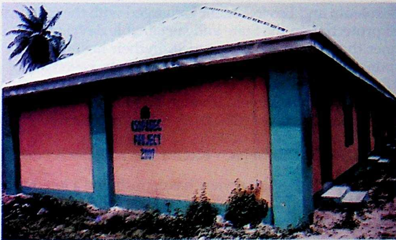
Renovated Town School Oguta Classroom by ISOPADEC
