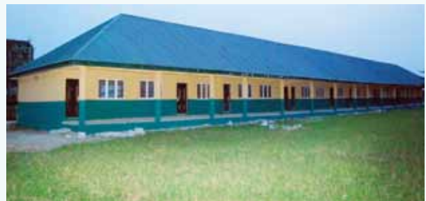
Renovated six class rooms block with two staff office at Army Day Secondary School,Effurun ,Uvwie L.G.A.
