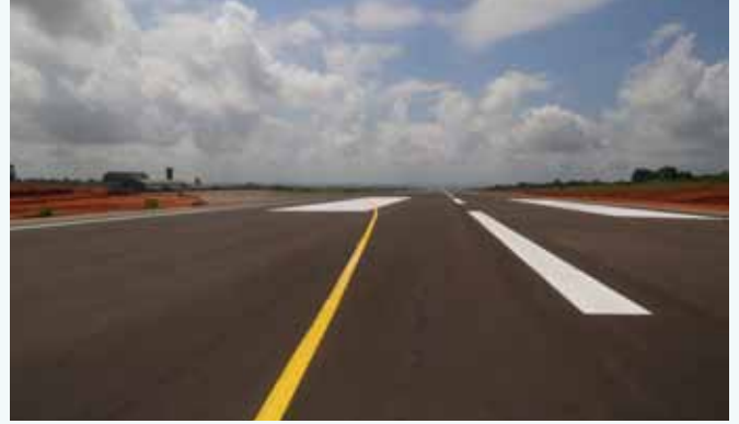
Reconstructed runway at Asaba airport expanded to 3.4km long and 45 metres wide with associated taxi ways.
