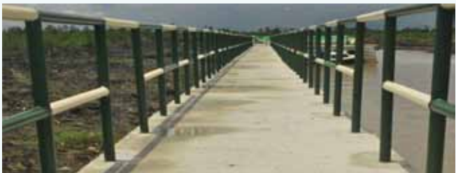
110 meters concrete landing jetty at Aji-Gba community in Warri South L.G.A
