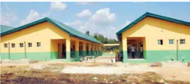
Block of Class Rooms Block at Kokori Mixed Secondary school, Kokori, Ethiope East.
