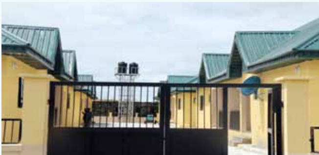
Housing Estate for Teachers and Medical Doctors at Okerenkoko Community, Warri South West L.G.A.
