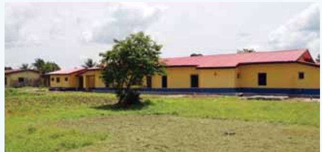
Central Hospital Ughelli, Ughelli North LGA
