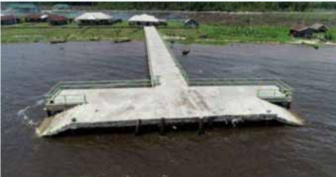
167meters Length with 88m Width Landing jetty at Oboghoro, Warri North L.G.A
