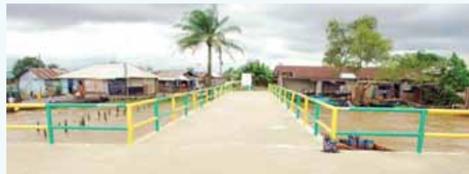
Concrete landing jetty at Naifor Island , Warri South L.G.A.
